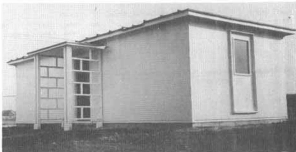
Figure 4.—Sandwich experimental unit as re-erected in 1968. (M 135 634-3)
