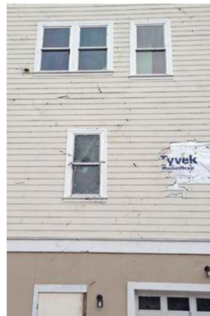
THE ONLY DAMAGE TO THE MGO SIP HOME WAS TWO CRACKED IMPACT WINDOWS AND DAMAGE TO THE VINYL SIDING
