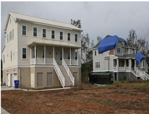
THE ONLY DAMAGE TO THE MGO SIP HOME WAS TWO CRACKED IMPACT WINDOWS AND DAMAGE TO THE VINYL SIDING
